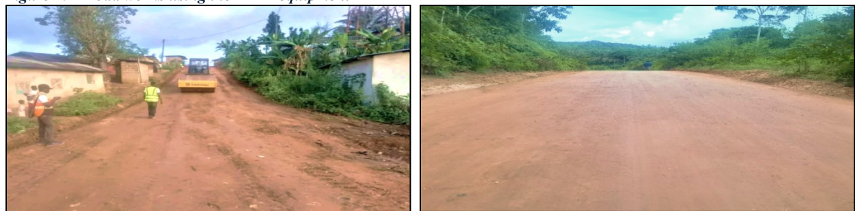
Figure 29 - Road works using the DRIP equipment
