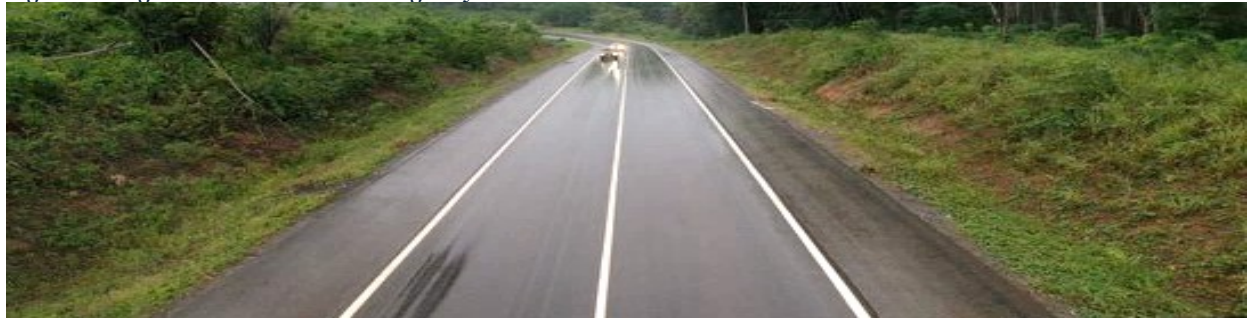
Figure 28 - Agona Nkwanta - Tarkwa Highway
