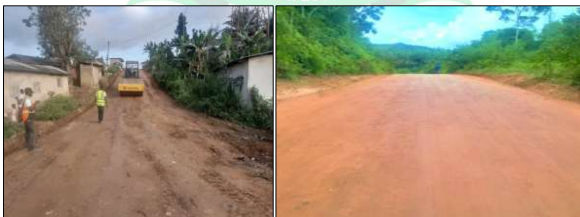
Figure 19 – Road works in some communities using the DRIP equipment
